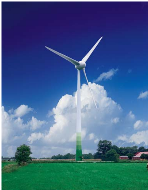
Application Example Wind Turbine
